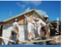
Repairing the field station on Round Island
